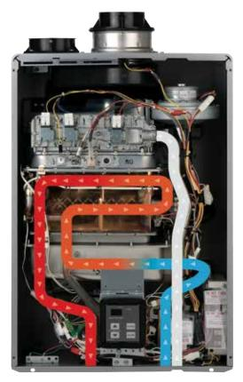
HOT COLD GAS WATER WATER INLET OUTLET INLET
