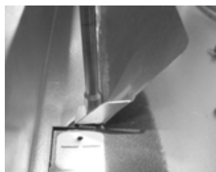
Step 2: Secure all three of the screws to the up-right positioned heat shield - one (1) at both ends and one (1) in the center.
