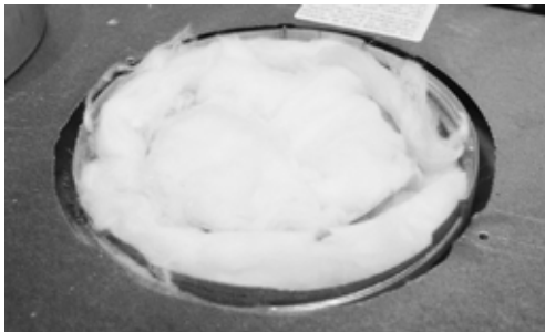
Step 3: Remove insulation from inside flue pipe.
