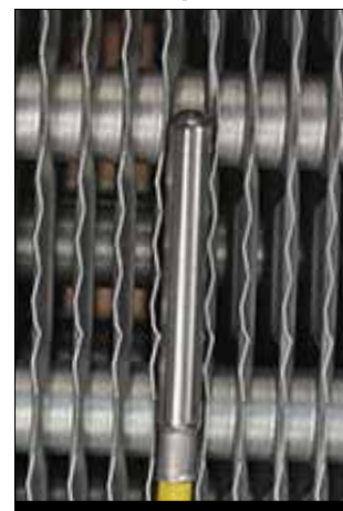
Figure 5 - Option 2: Sensor Positioned Parallel to Evaporator Fins
