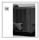
The outdoor fan motor has sleeve bearings and is inherently protected. The motor is totally enclosed for maximum protection from weather, dust and corrosion. (20) Access to the outdoor fan is made by removing four fasteners from the fan grille. The outdoor fan can be removed from the fan grille by removing 4 fasteners in the rare case outdoor fan motor fails.
