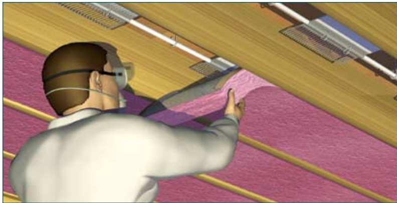
R-12 fiberglass insulation
