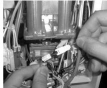
Attach the cable tie bracket to the bottom of the water heater cabinet using the existing screw. Pull all of the excess cable up into Unit 2's cabinet, and then secure it tightly to the bracket using the cable tie.
