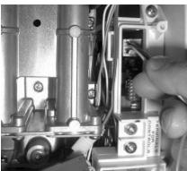
Remove the protective cap from the 2 pin connector marked "MS" (located in the middle of the Continuum water heater wiring harness).
