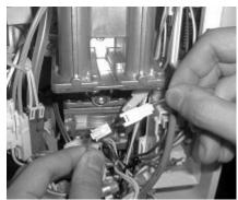
Attach the cable tie bracket to the bottom of the water heater cabinet using the existing screw. Loosely secure the cable tie through the bracket and around the communication cable. DO NOT TIGHTEN THE CABLE TIE AT THIS TIME -- the communication cables from the other water heaters must be secured by this cable tie.
