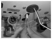
Route the 5 pin connector of Communication Cable B through the 10) cable tie, installed in step 8, and plug it into socket 2 on Master Communication PCB.
