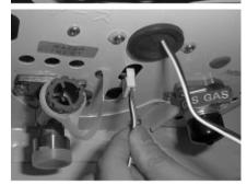
Connect the 4 pin connector from 12) Communication Cable B to the 4 pin socket located at the top of the water heater Unit 2's PCB.
