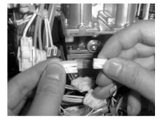
Connect the 2 pin connector from Communication Cable B into the 2 pin 14) connector marked "MS".
