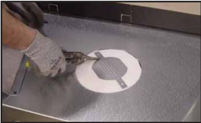
Figure 9.2 Cut the seal cap strap across the rectangles next to the disk.
