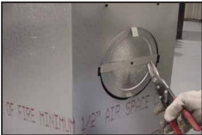
Figure 9.9 Cut the metal retaining band and fold the sides out.
