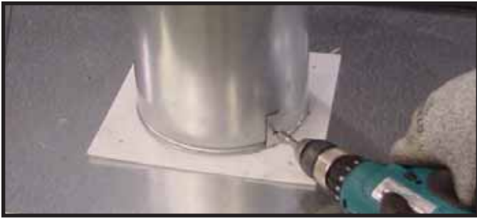
Figure 9.7 To attach the first section of vent pipe, make sure to use the fiberglass gasket in the manual bag to seal between the first vent component and the outer fireplace wrap. Use 2 self tapping screws to secure the gasket to the outer wrap.
