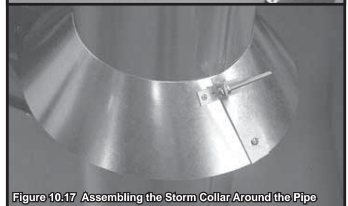
Figure 10.16 Assembling the Storm Collar
