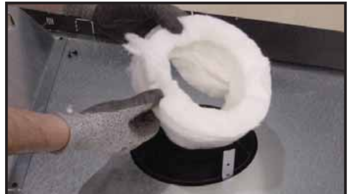
Figure 9.6 Remove the insulation from the outer vent pipe. For rear venting there is no insulation in the outer vent pipe.
