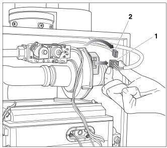
Fig. 81 Removing the connectors from the fan
