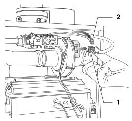
• Remove both the fan unit power supply cord plug [1] and the fan unit tacho cable plug [2].
