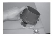
Place the orange rubber ring on the bottom of the exhaust collar, and align the exhaust collar on top of the aluminum mounting flange.
