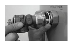
Insert O-ring gasket before installing T&P valve to ensure a tight seal.
