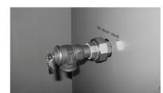
Install the T&P Valve on the side of the unit and tighten.
