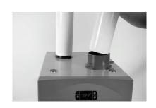
Insert the PVC vent pipe into the Exhaust Collar but do not use glue to seal the connection, the collar acts as a coupling and forms an airtight seal.
