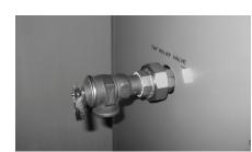
Install the T&P Valve on the side of the unit and tighten.
