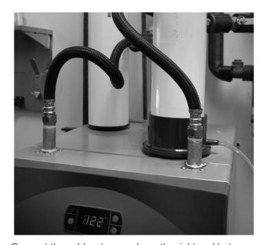
Connect the cold water supply on the right and hot water outlet on the left. Do not reverse the water connections as the unit will not work. Make sure the pipes are tightened to avoid leaks.
