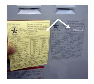
The GU32 can only be down-rated to GU28, which limits maximum input to 199,000 BTUs/HR.
