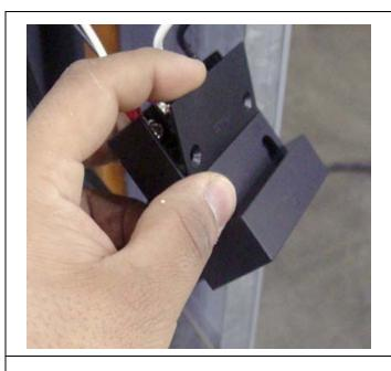
Remove four Phillips head screws to loosen the wiring
