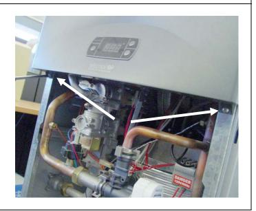
Remove the 4 screws securing the LED Display to the Front Panel.
