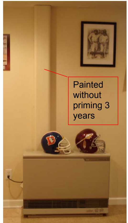
Painted Vent Cover/Basement Installation
