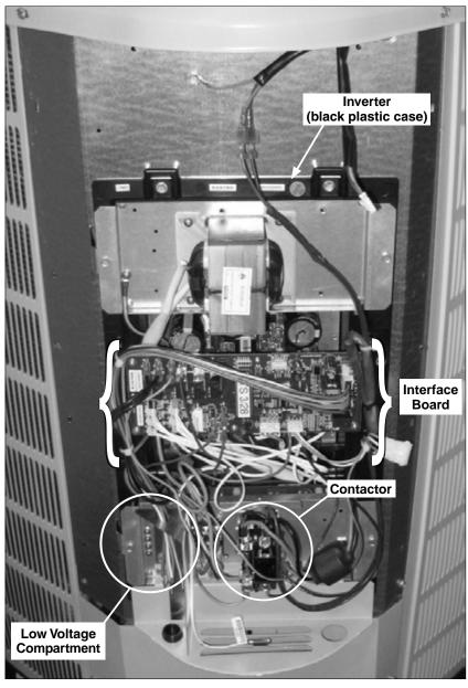
Figure 2. Heat Pump Control Panel (Cover Removed)
