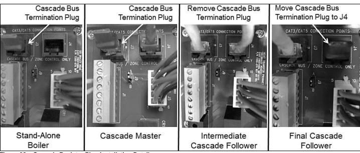
Figure 32 – Cascade Resistor Plug Installation Detail
