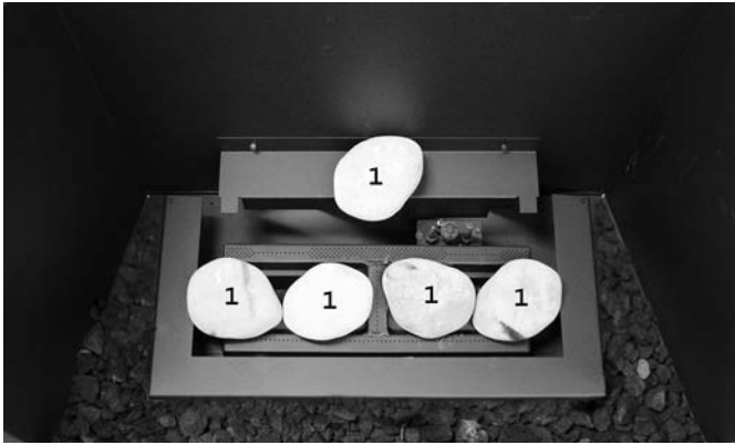
STEP 5: Place rocks #1 onto the burner as shown. Do not place rocks directly onto the burner tubes.
