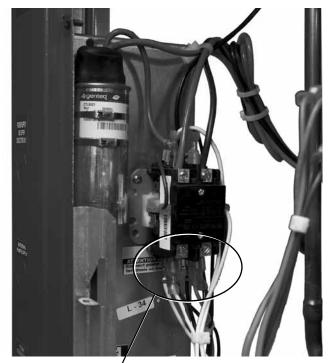
Unit Power Supply (see electrical tables 5a - 5b for minimum circuit amps and maxiumum breaker size)
