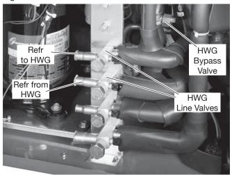
Figure 21b: Remote HWG Module
