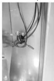
Discharge Air Sensor
