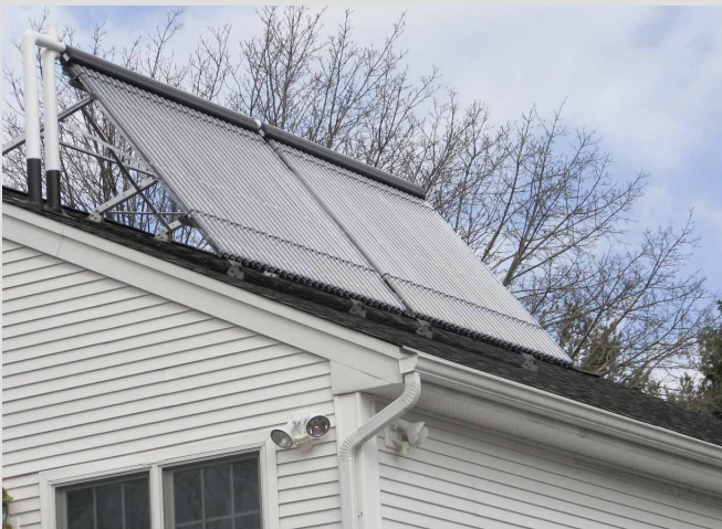
Vitosol 300 – vacuum tube solar collectors
