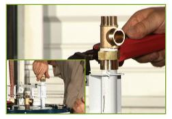
10. Put Teflon tape on the ¾" nipple thread and attach the ¾" Flange Adaptor to the ¾" nipple. Tighten the Flange Adaptor with your adjustable wrench with enough force to prevent leakage. Put Teflon tape to all the threads of the 'T' Adaptor. Attach the 'T' Adaptor to the Flange Adaptor and tighten it using a pipe wrench.
