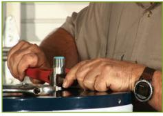
4. On most electric (or gas) water heaters, the inlet and outlet connections consist of two ¾" nipples extending from the top of the tank. First, disconnect the hot outlet pipeline from the nipple, then using your pipe wrench, remove the ¾" nipple extending from the hot outlet port of the water heater.
