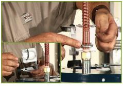
8. Now attach the forked mounting bracket to the cold inlet nipple. To do this, first remove the U-Bolt, and place the fork onto the nipple. Now screw the U-Bolt back in place, using the provided washers to keep the bracket tight. Make sure there is a slight slope toward the front of the water heater.
