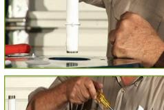
and Cold ports. The stopper for the Hot port must be removed to allow clear passage. It is also common to find an Anode Rod to help prevent corrosion of the water tank. This should be removed as well and reinstalled in the Cold Port side. To do this, remove the Cold Inlet Pipe and nipple and attach the Anode Rod to the stopper within the port. Because you will be submerging copper tubing into the tank, it is important that this rod be replaced once every 2 years.
