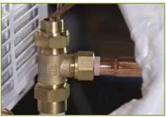
17. This is a good time to check for leaks in the new connections.
