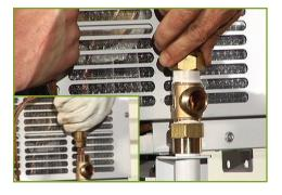
13. Apply teflon tape to the threads on the exposed end of the outlet nipple previously installed. Screw the brass female adaptor onto the nipple and tighten securely. Tighten all adaptors.
