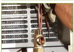
**USE CAUTION** during the immersion process to ensure that no crimping of the coil or thermostat capillary takes place, including the section from the insertion nipple to the back of the AirTap $^{\text{TM}}$ . At no point should you allow the coil to curve with more than a 2" radius.
