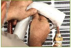
15. Find the copper tube that extends from the back of the AirTap™. Place the foam insulation pipe around this tube. You may also cover the hot outlet pipe coming out of the tank.
