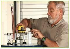
9. Make sure the two brackets are level with one another by placing your level across the two. Be sure to check that there is a slight slope to the front of the water heater. This slope is needed because it allows easy drainage of any condensation that may form on the AirTap™ unit. To test this slope, pour a small glass of water over the top of the unit and follow the path of the water flow.
