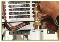
16. You can now reconnect the hot water line on the side, and turn on the cold water supply to the water heater. Once the air has escaped from the system, go ahead and turn off the faucet(s) that you had turned on.
