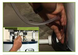
14. Now attach the drain hose to the AirTap™, and feed it through your drain line.
