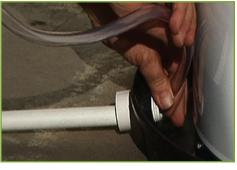
3. Make sure that the unit has access to a drain, so that the condensate produced by the AirTap™ can escape. During periods of high humidity, the level of condensate can be up to 1 quart per day.
