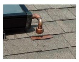
•Using a wood bit the same size as your pipes, drill a hole in the center of a shingle below where the bottom corner of the collector will be and in the opposite corner where the collector outlet will be.
