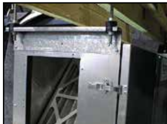
Figure 3. Unit hung from ceiling using optional hanging bracket kit, 45EVHB. To install hanging bracket, identify the corners of unit you wish to hang it from. Remove existing screws from unit pan. Attach hanging bracket to unit using screws provided with the hanging bracket.
