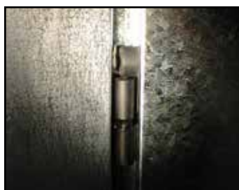
Figure 8. Rubber Door Keeper installed on Filter Access (small) Door.
