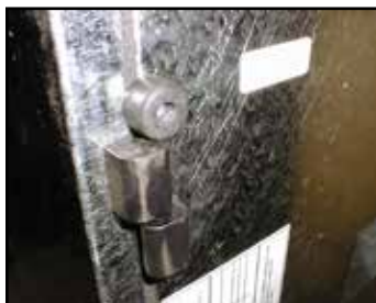
Figure 7. Rubber Door Keeper installed on Blower Access (large) Door.
