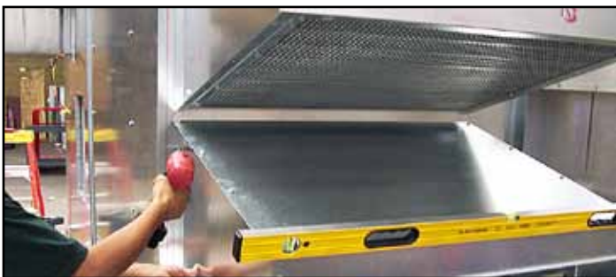
Figure 2 - Install Center Hood
