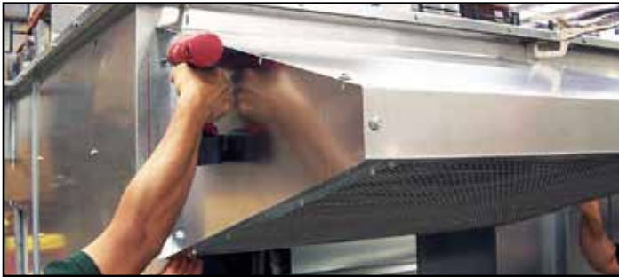
Figure 1 - Install Top Hood First
