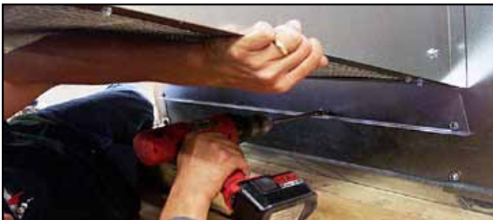
Figure 3 - Install Bottom Hood and Plate
