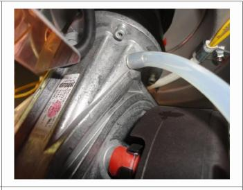
Connect the other end of the air tube (with brass orifice) to the Air Pressure Switch port marked with (H).
